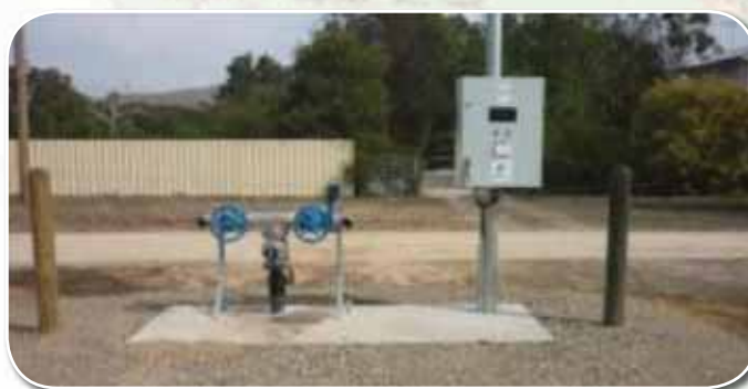
Figure 47: An electronic swipe card stand pipe. Source: https://vicwater.org.au/
