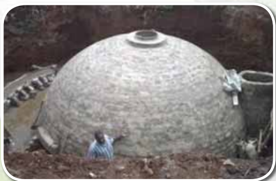
Figure 48: A biodigester under construction. Source: http://www.thebiooasis.com/biodigester/
