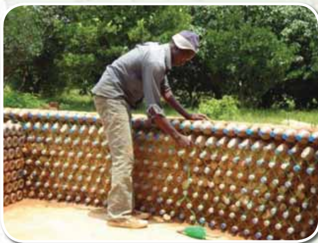
Figure 73: A plastic bottle housing unit under construction. Source: http://www.ru-screw.com/end-homelessness-using-plastic/
