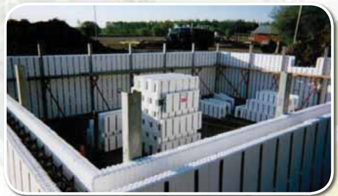
Figure 70: An EPS housing unit under construction. Source: http://sherryvsthebackcountry.ca/?p=2271
