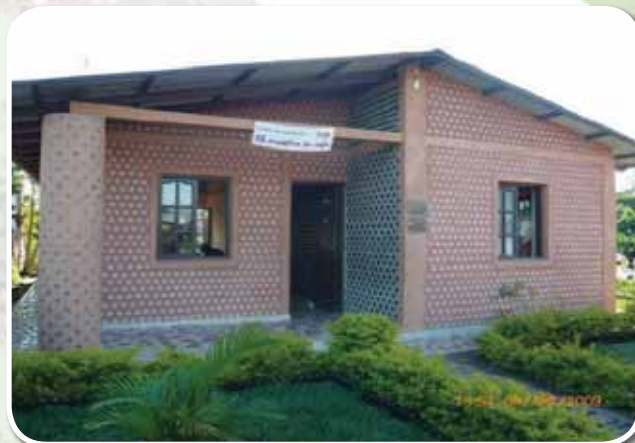
Figure 72: A housing unit constructed from plastic bottles. Could plastic bottle housing be the solution to Clarendon's low income housing needs? Source: http://www.instructables.com/id/New-Innovation-in-Construction-using-Waste-Plastic/
